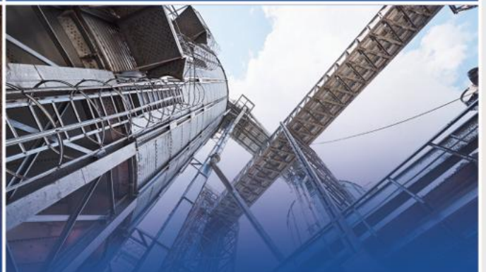
INDUSTRIAL & INFRASTRUCTURE SCADA, PROCESS CONTROL, AND INDUSTRIAL IOT SOLUTIONS.
